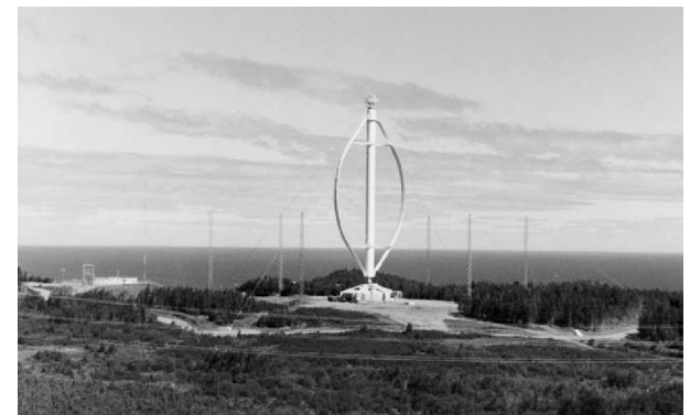
Darrieus configuration Canada, 1987 4000 kW, Höhe 100m D = 64m
